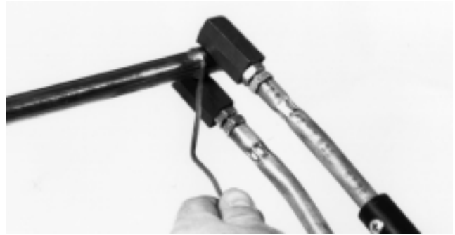
Figure 6 – Soudage du raccord
